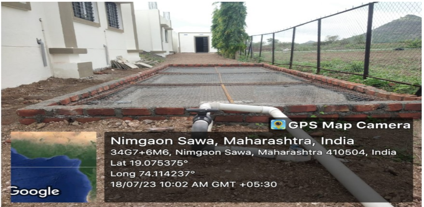
Tank Constructed for water conservation
