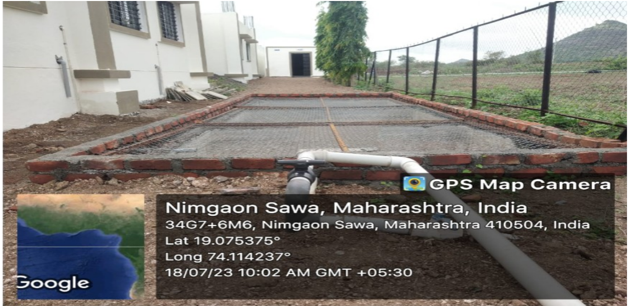
Tank Constructed for water conservation
